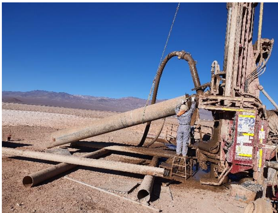
Figure 2 – Andinor construction of a 400m production well.
