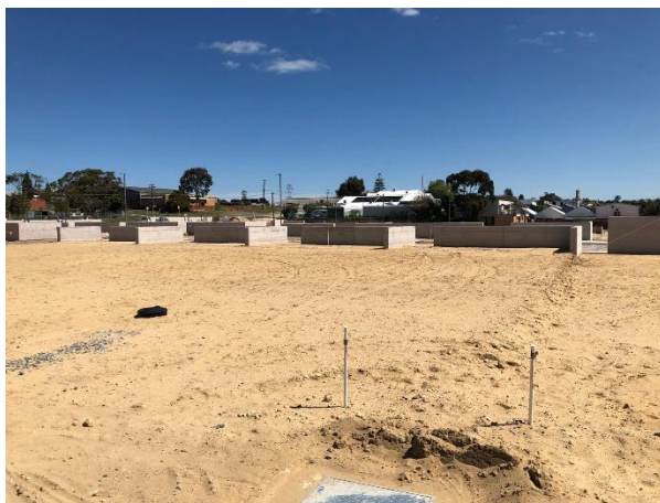
Cleared and prepared site at Knutsford East Village.
