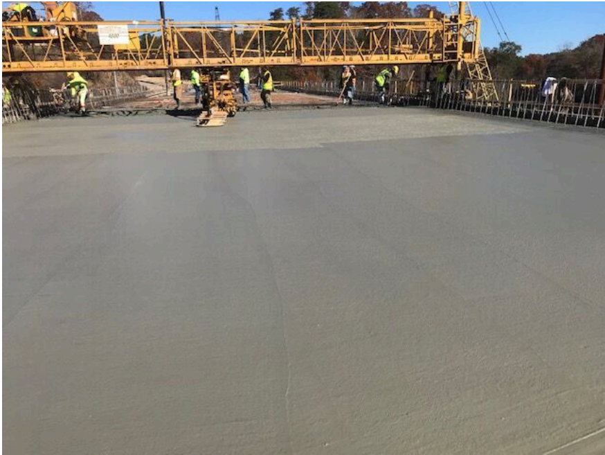
Figure 1. Bridge over Little River showing freshly lain concrete bridge decking
