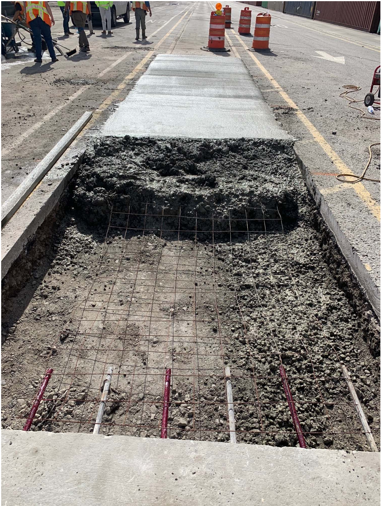
Figure 1. EdenCrete®- enriched concrete being poured at Garden City Terminal, Port of Savannah
