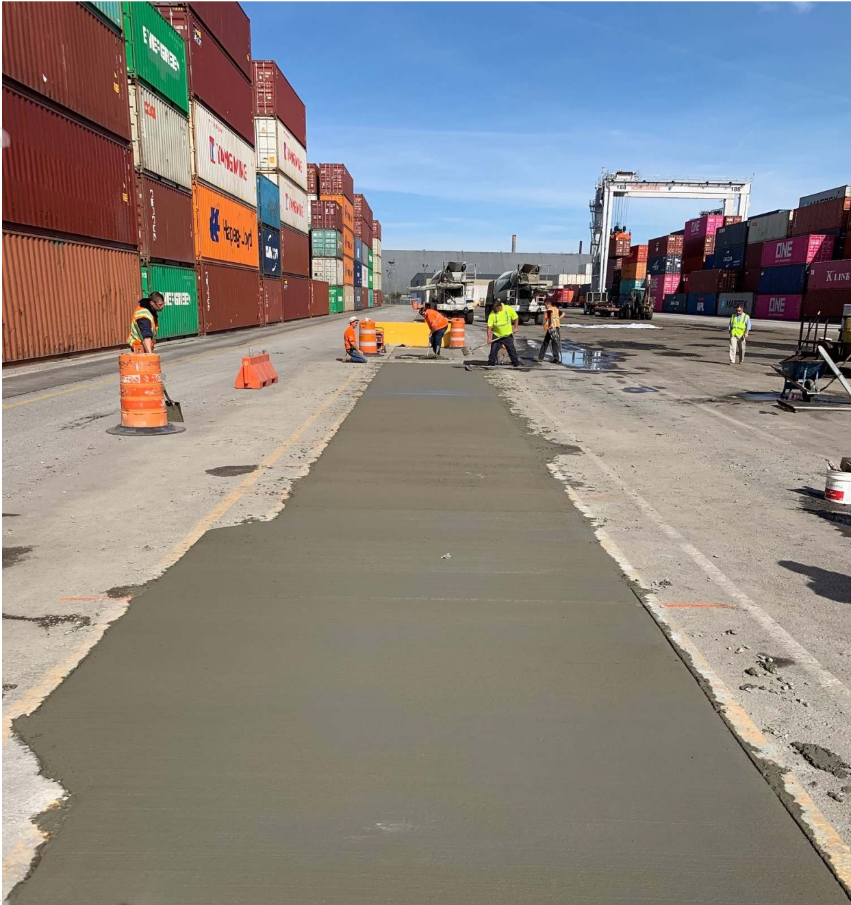
Figure 2. EdenCrete®- enriched concrete being poured at Garden City Terminal, Port of Savannah
