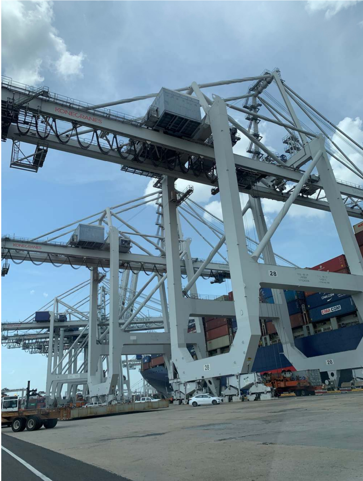
Figure 3. Some of approximately 30 ship-to-shore cranes currently operating at Port of Savannah
