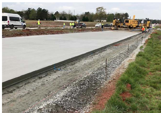
Figure 1. Completed section of highway with added EdenCrete
