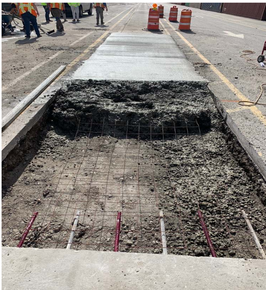
Figure 1. EdenCrete®- enriched concrete being poured at Port of Savannah
