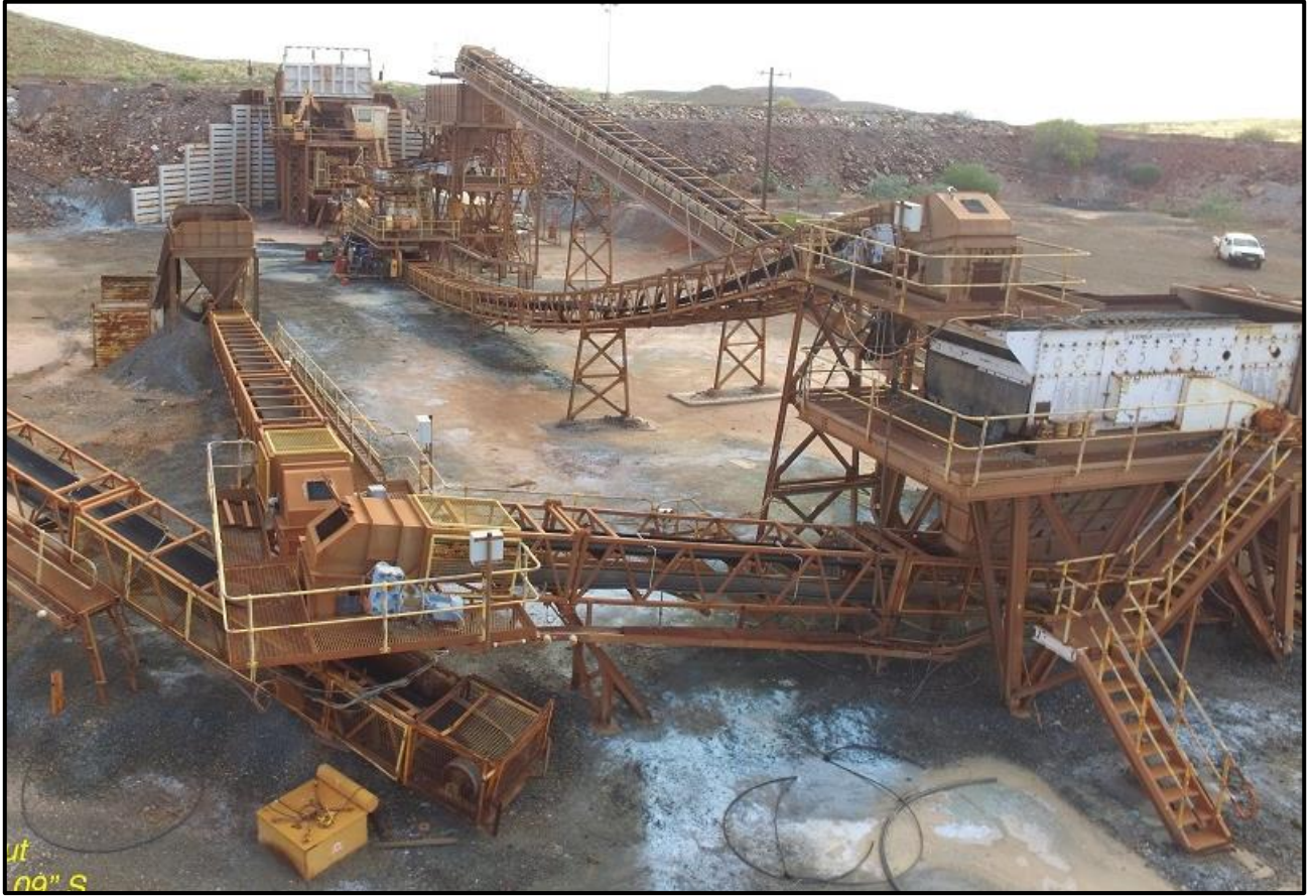
Figure 2: Existing Crushing Infrastructure at the Whim Creek Project
