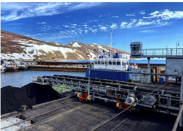
Belt conveyor loading of TIG's 500t barge
