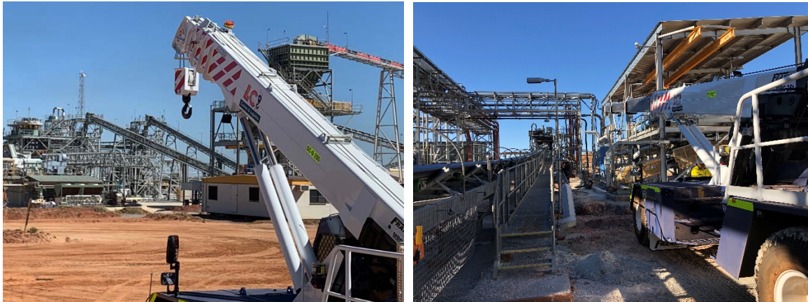
Figure 4 – LC Cranes MRC 25T Franna on Altura’s Pilgangoora Site
