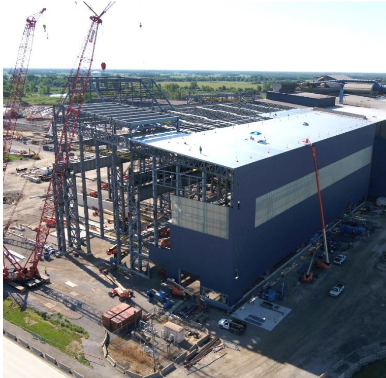
Melt shop building cladding underway
