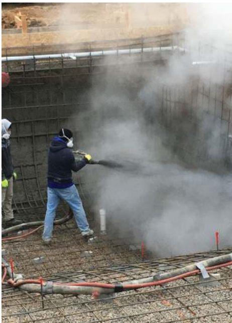
Figure1 Shotcrete trial without added EdenCrete®
