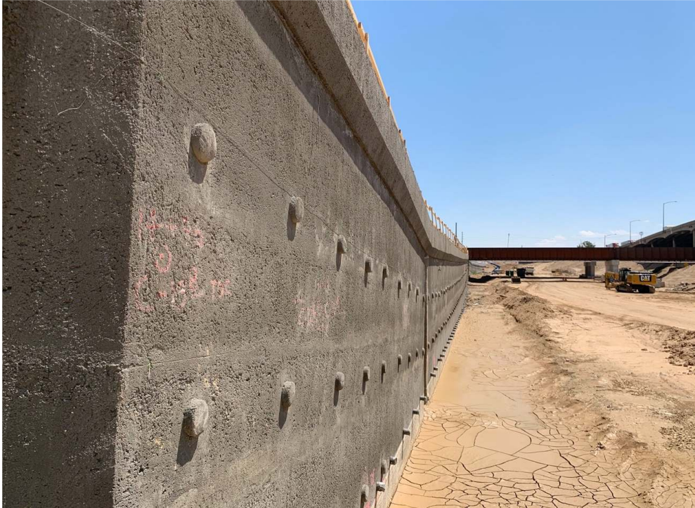
Figure 8. Retaining wall along Central 70 project constructed using EdenCrete® shotcrete.
