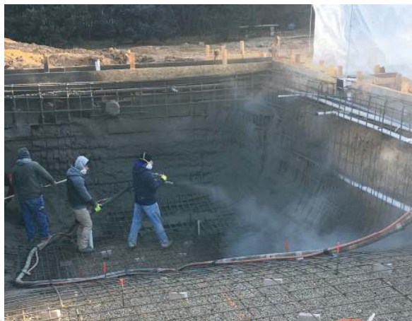
Figure 2 Shotcrete trial with added EdenCrete®
