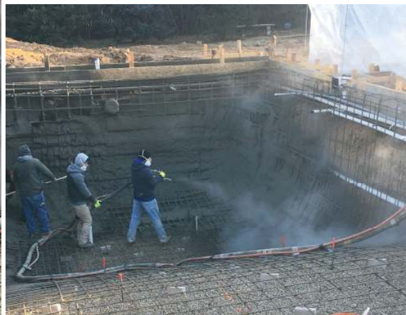
Figure 2 Shotcrete trial with added EdenCrete®
