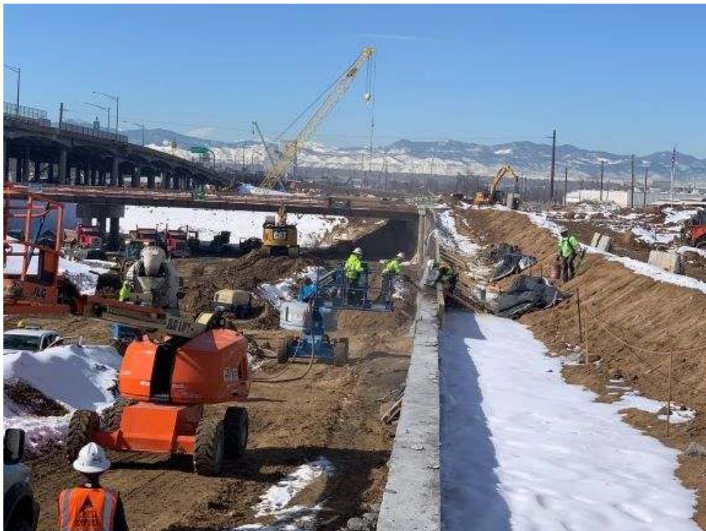
Figure 9. Retaining wall being constructed along Central 70 project using EdenCrete® shotcrete
