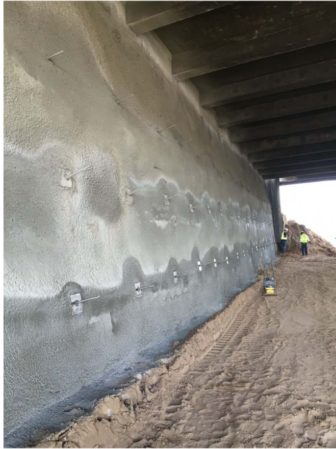
Figure 10. Retaining wall constructed under bridge using EdenCrete® on Central 70 project.
