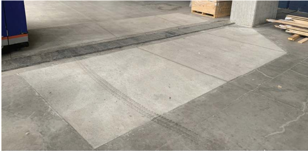
Figure 2. Interior Corridors- 4-inch-thick overlay on suspended slab
