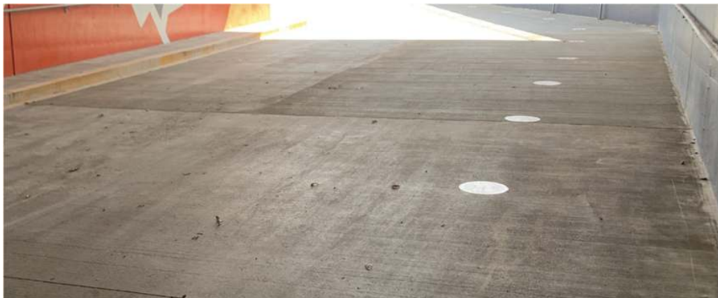
Figure 7. Freight Access Ramps- 8 inch thick slab on grade- 5000psi (35MPa) structural concrete
