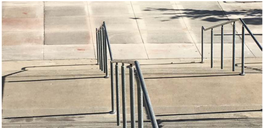
Figure 4. Perimeter Facilities - 5- 6-inch-thick, full-depth slab repair.
