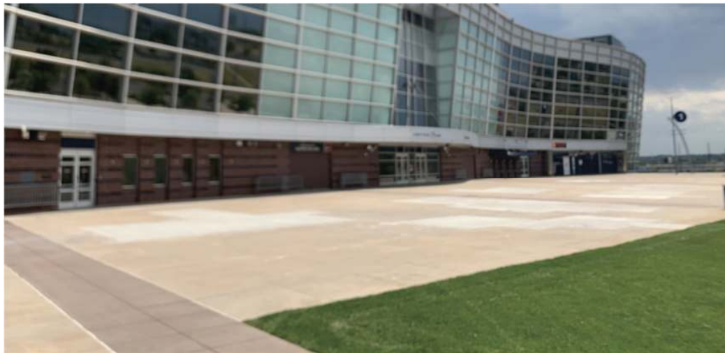
Figure 3. Exterior Corridors - 5-6-inch-thick full-depth slab
