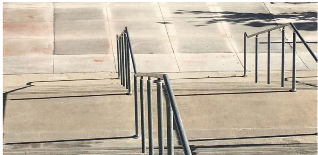
Figure 4. Perimeter Facilities - 5- 6-inch-thick, full-depth slab repair.
