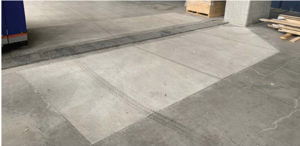
Figure 2. Interior Corridors- 4-inch-thick overlay on suspended slab
