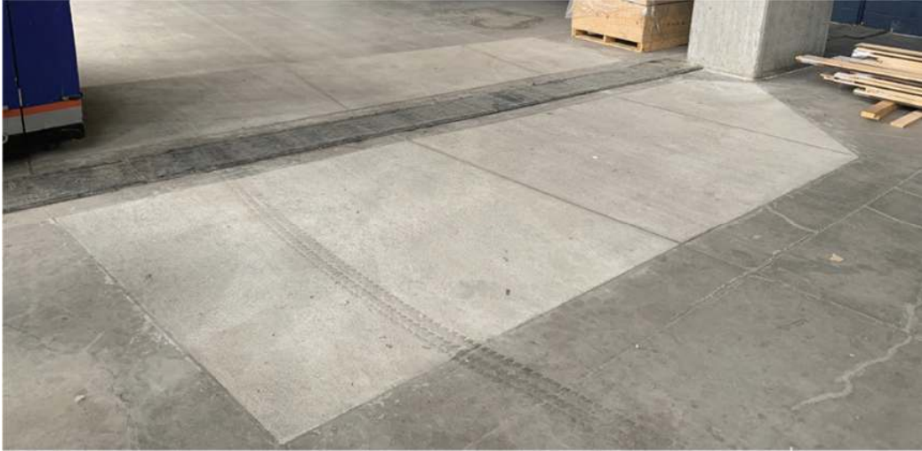
Figure 2. Interior Corridors- 4-inch-thick overlay on suspended slab
