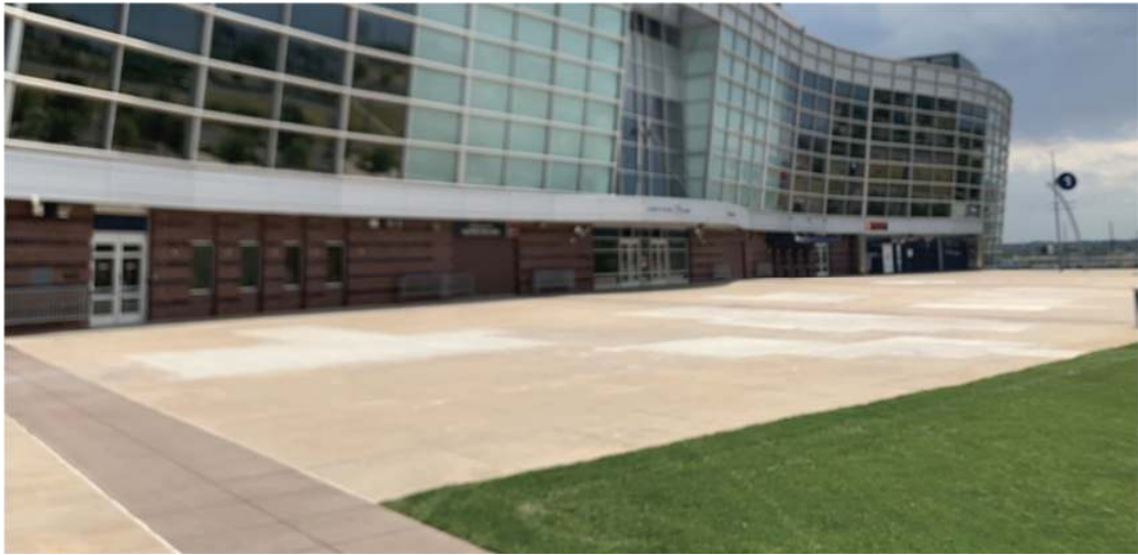
Figure 3. Exterior Corridors – 5-6-inch-thick full-depth slab
