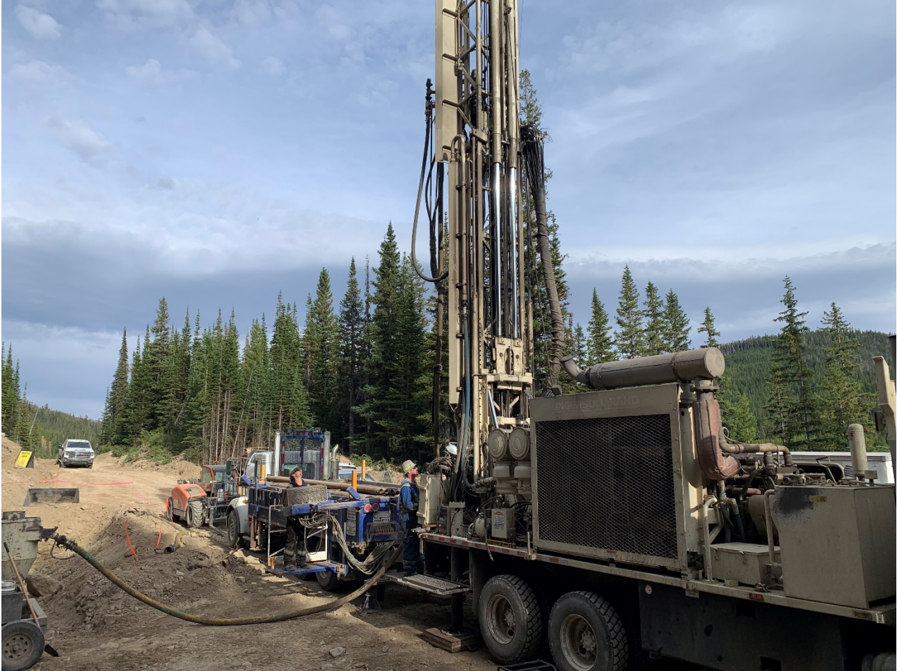
Large diameter drill rig at Chinook Vicary, 21 September 2020
