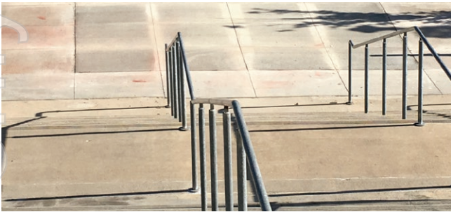
Figure 7. Perimeter Facilities - 5- 6 inch thick, full-depth slab repair.
