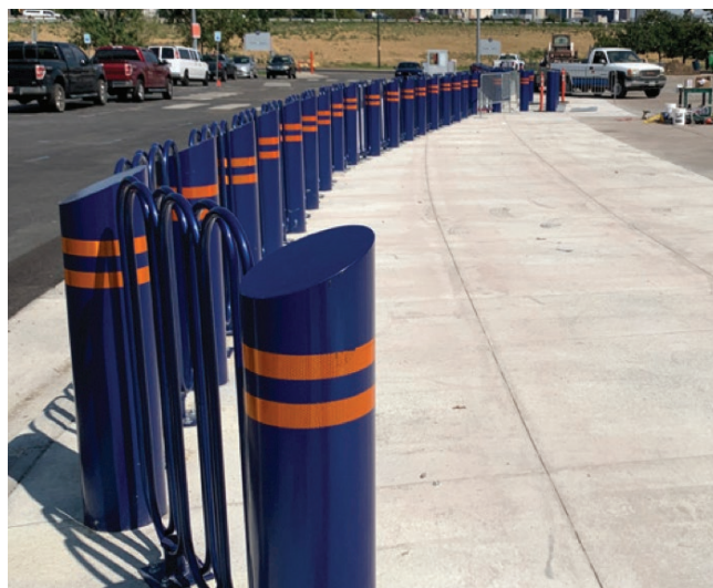
Figure 13. Steel Bollard security Screening Areas - 6 inch thick full-depth slab.
