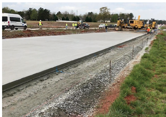
Figure 1. Completed section of highway with added EdenCrete®.
