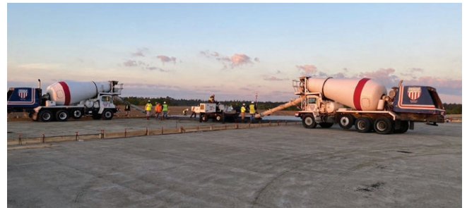
Figure 15. 200,000 square foot Industrial slab being poured.
