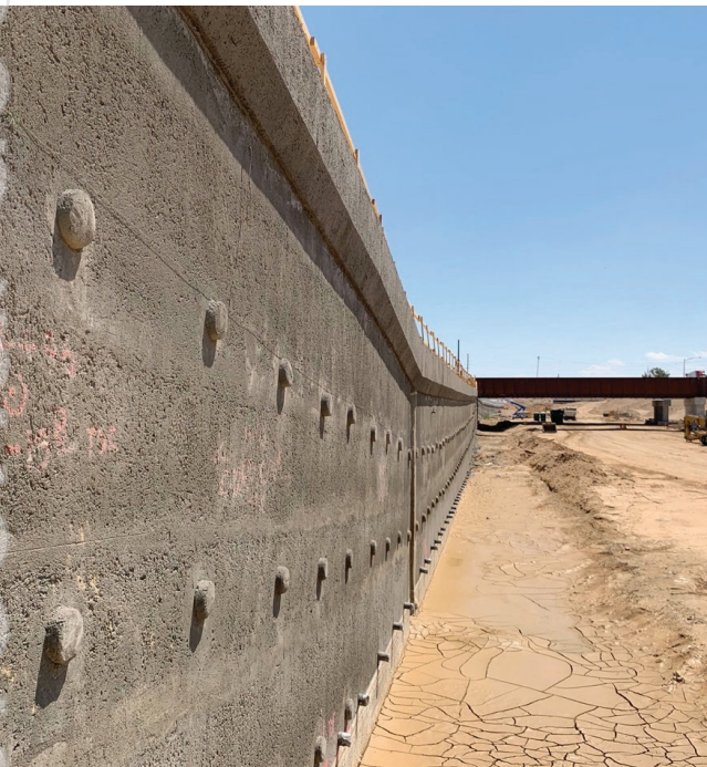
Figure 3. Retaining wall along Central 70 project constructed using EdenCrete® shotcrete.
