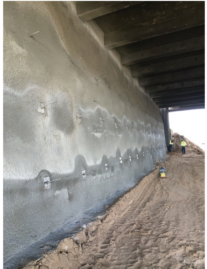
Figure 5. Retaining wall constructed under bridge using EdenCrete® on Central 70 project.
