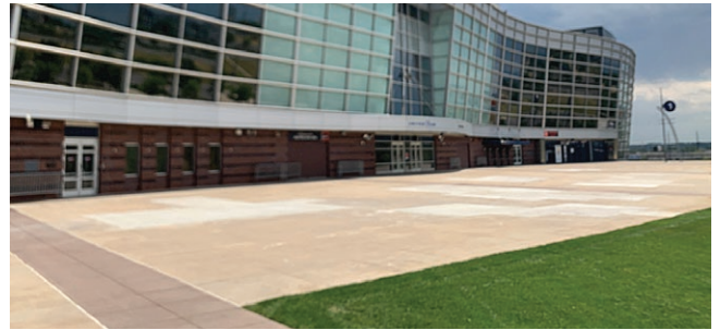
Figure 11. Exterior Corridors - 5-6 inch thick full-depth slab.
