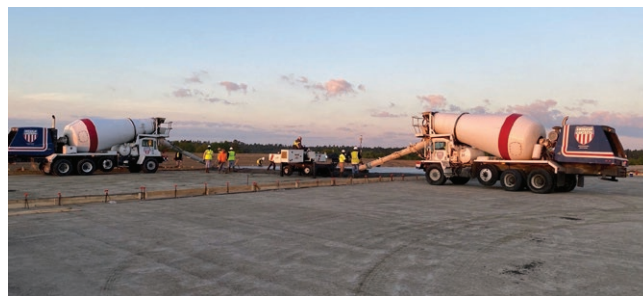
Figure 15. 200,000 square foot Industrial slab being poured.
