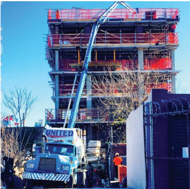
Figure 14. United Transit concrete being supplied to a construction project in New York.
