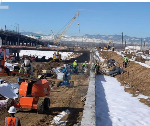
Figure 4. Retaining wall being constructed along Central 70 project using EdenCrete® shotcrete.
