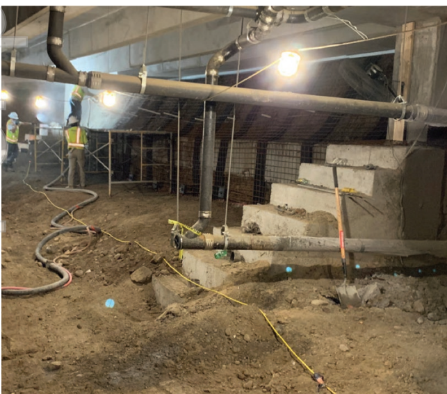
Figure 10. Centres for Health, Nutrition and Physical Therapy- EdenCrete® used in shotcrete for walls.
