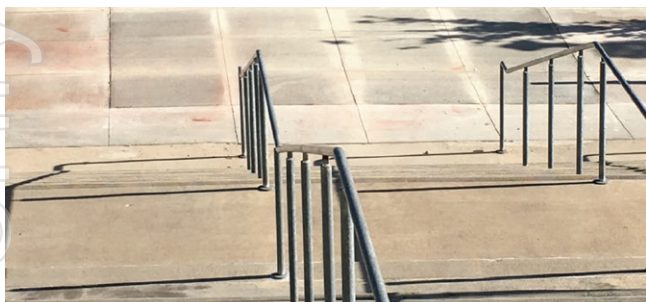
Figure 7. Perimeter Facilities - 5- 6 inch thick, full-depth slab repair.
