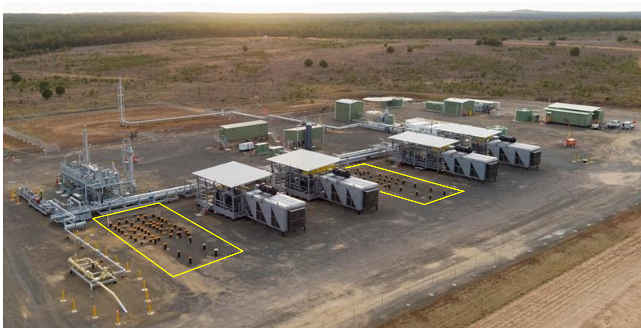
Roma North gas processing facility at 16 TJ/day (~6 PJ/year) nameplate capacity; footings in place (highlighted) ready for expansion to 24 TJ/day (~9 PJ/year)
