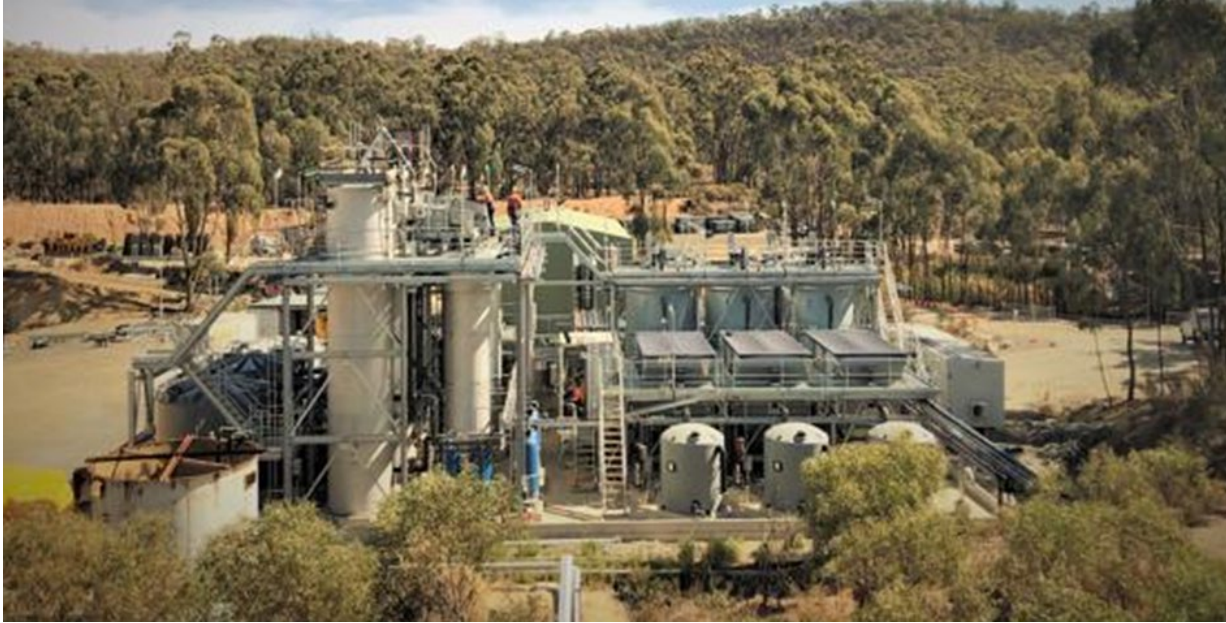
Clean TeQ plant installation at Fosterville Gold Mine, Victoria
