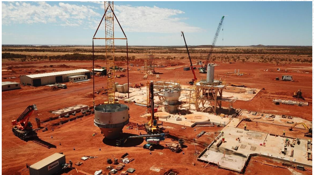
Figure 6: Process Plant site
