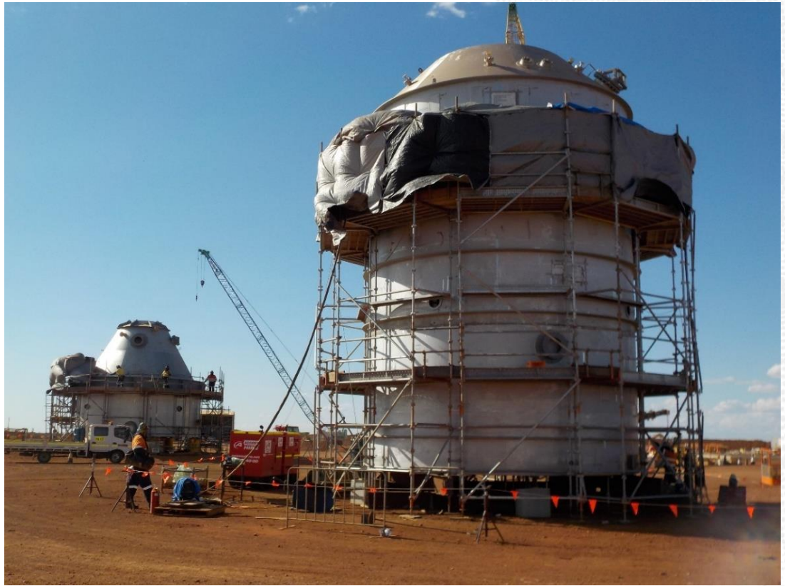
Figure 9: Tank fabrication
