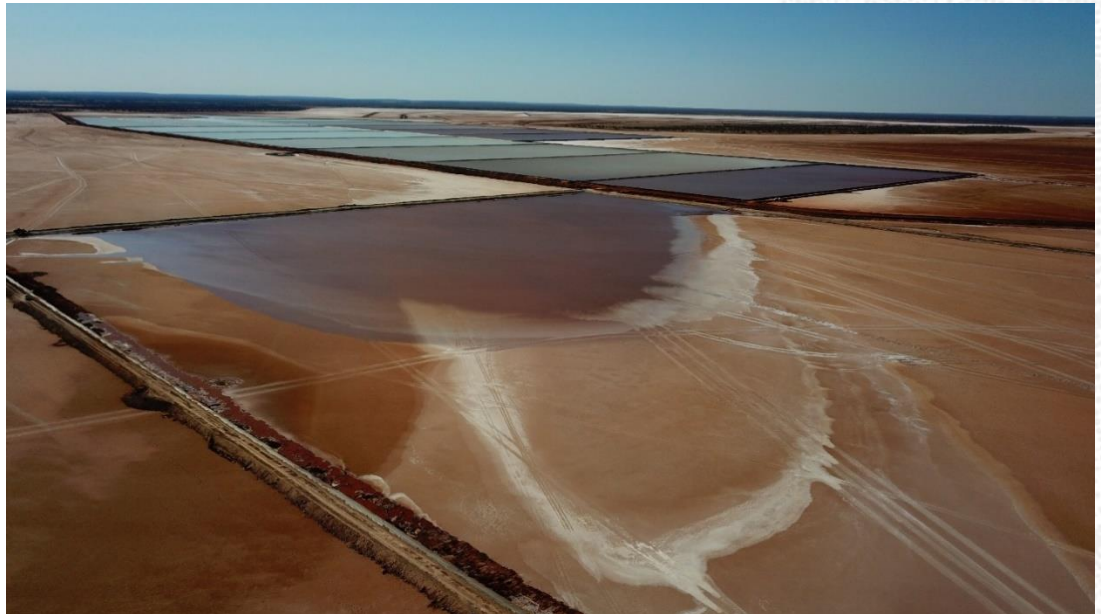
Figure 3: Commissioning of fourth pond train underway
