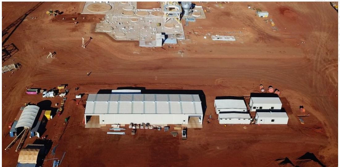
Figure 12: Lake Way warehouse, workshop, laboratory and ablutions
