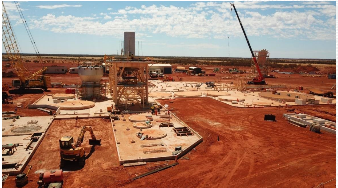
Figure 4: Process Plant site
