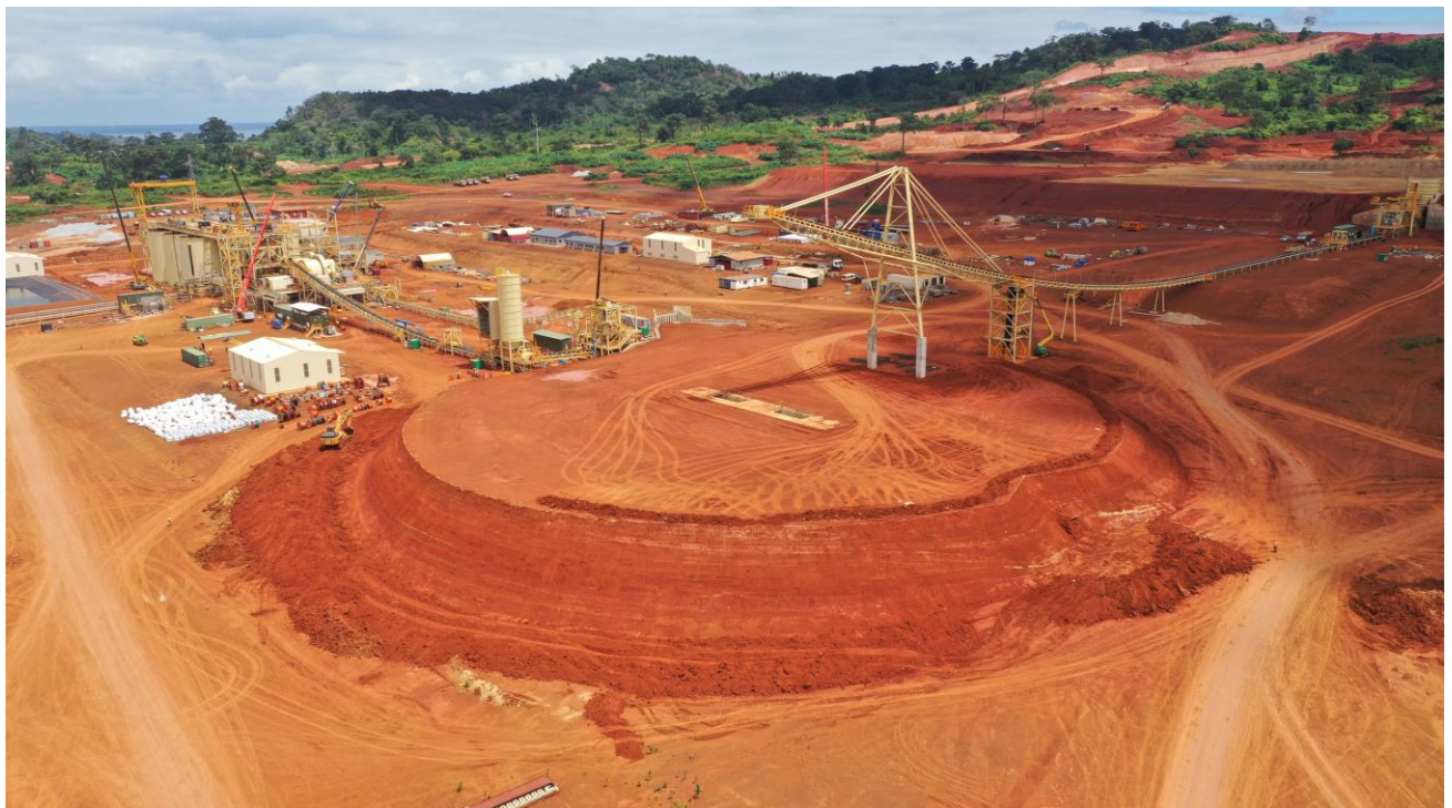
Crushed Ore Stockpile feed conveyor
