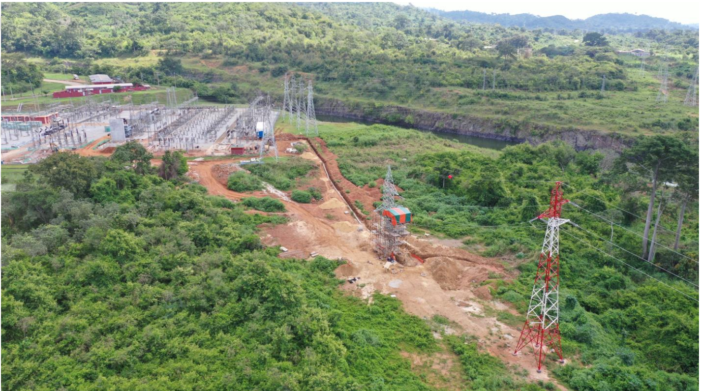
90 KV powerline installation
