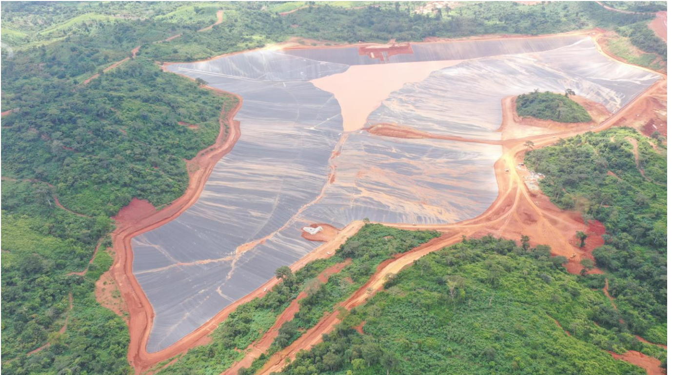
HDPE lined Tailings Storage Facility
