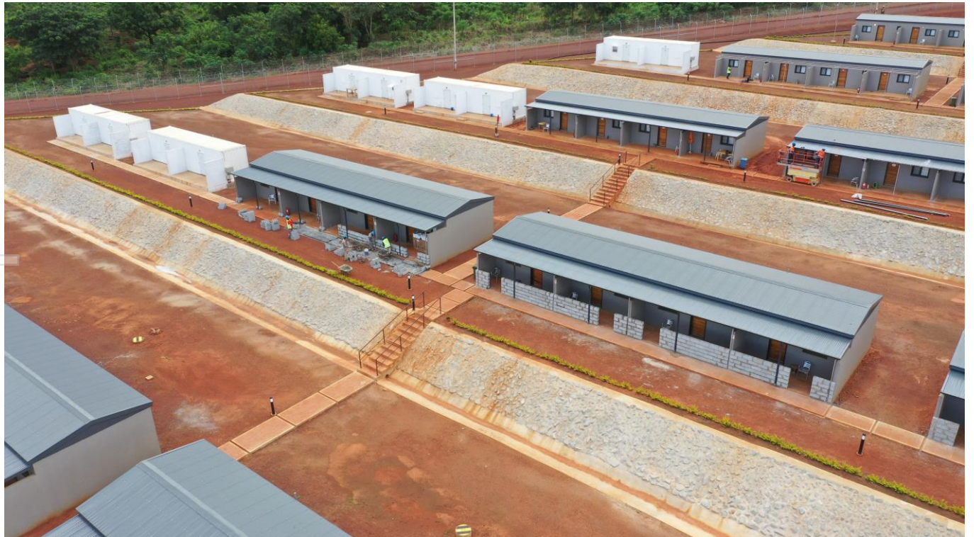
Permanent camp buildings
