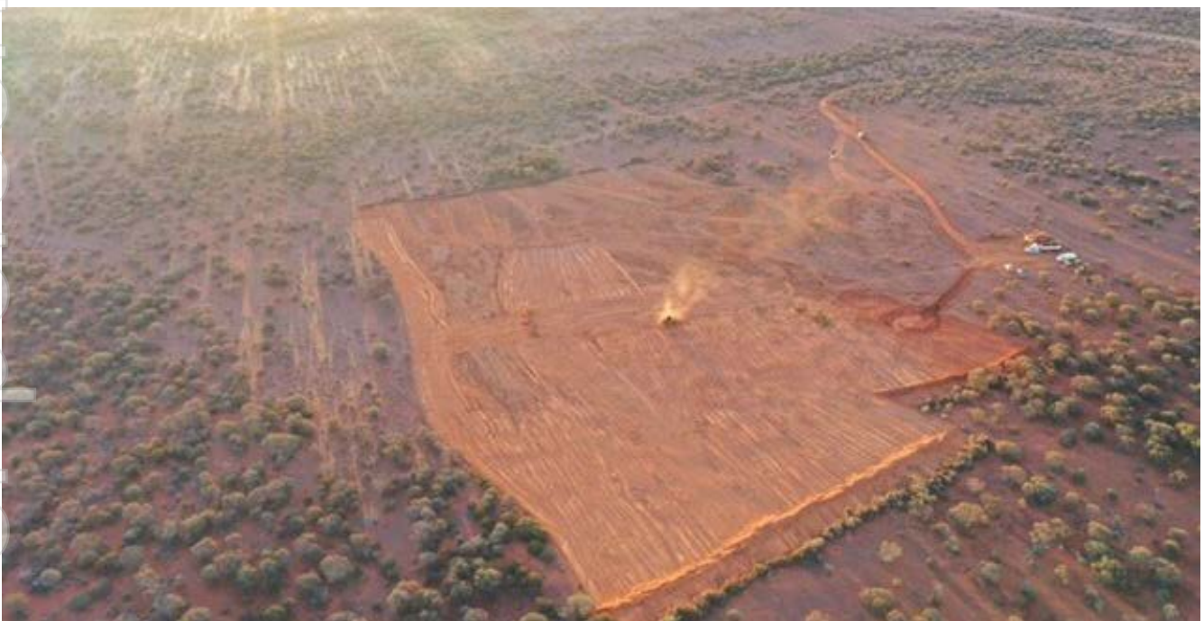
Figure 5 Site preparation for the new KOTH village and central facilities.
