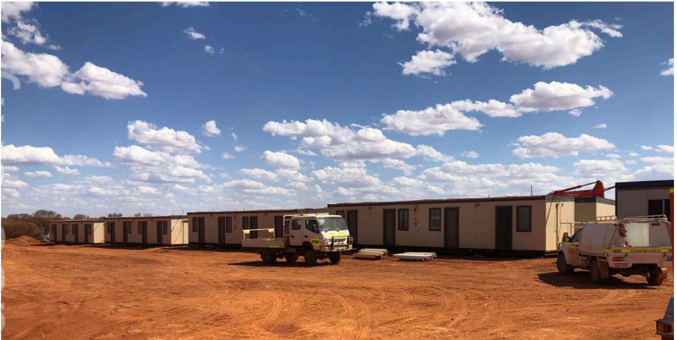
Figure 6 Construction of the KOTH village.
