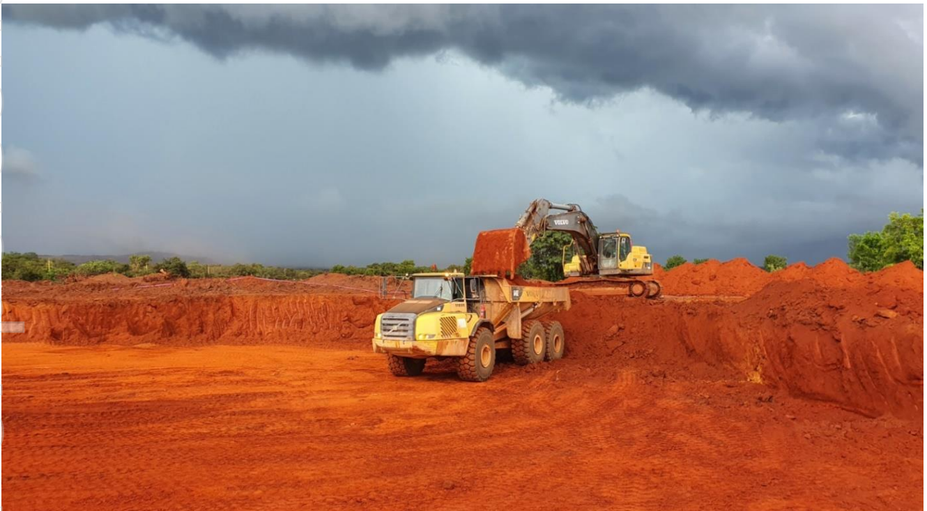
Figure 1: Establishment works at the Cashew mining operation
