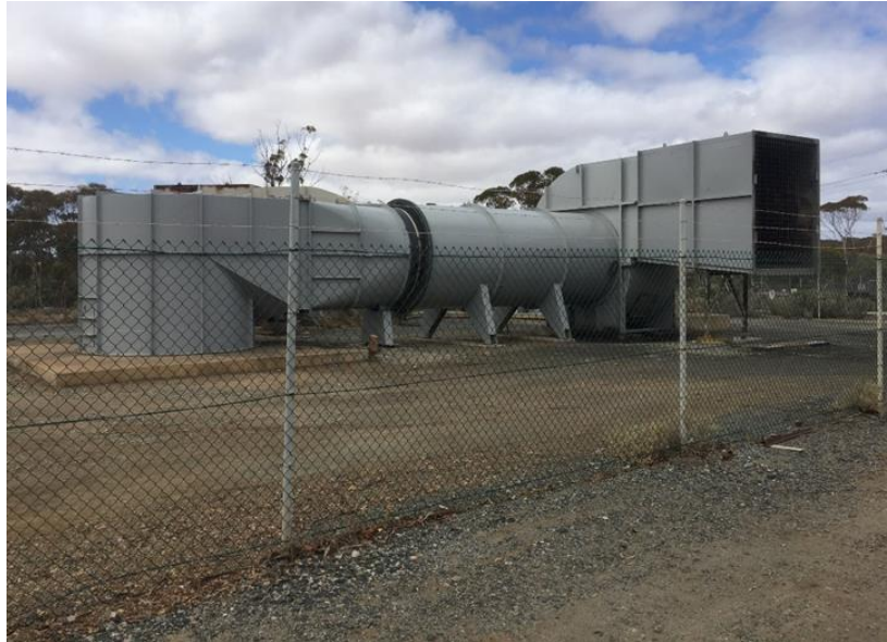
Northern Operations primary fan refurbished for the Otter Decline
