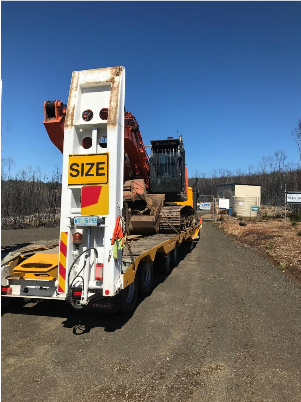
Figure 2 | Construction Equipment arrives at the Riley Mine Site on Tuesday 6 th October 2020
