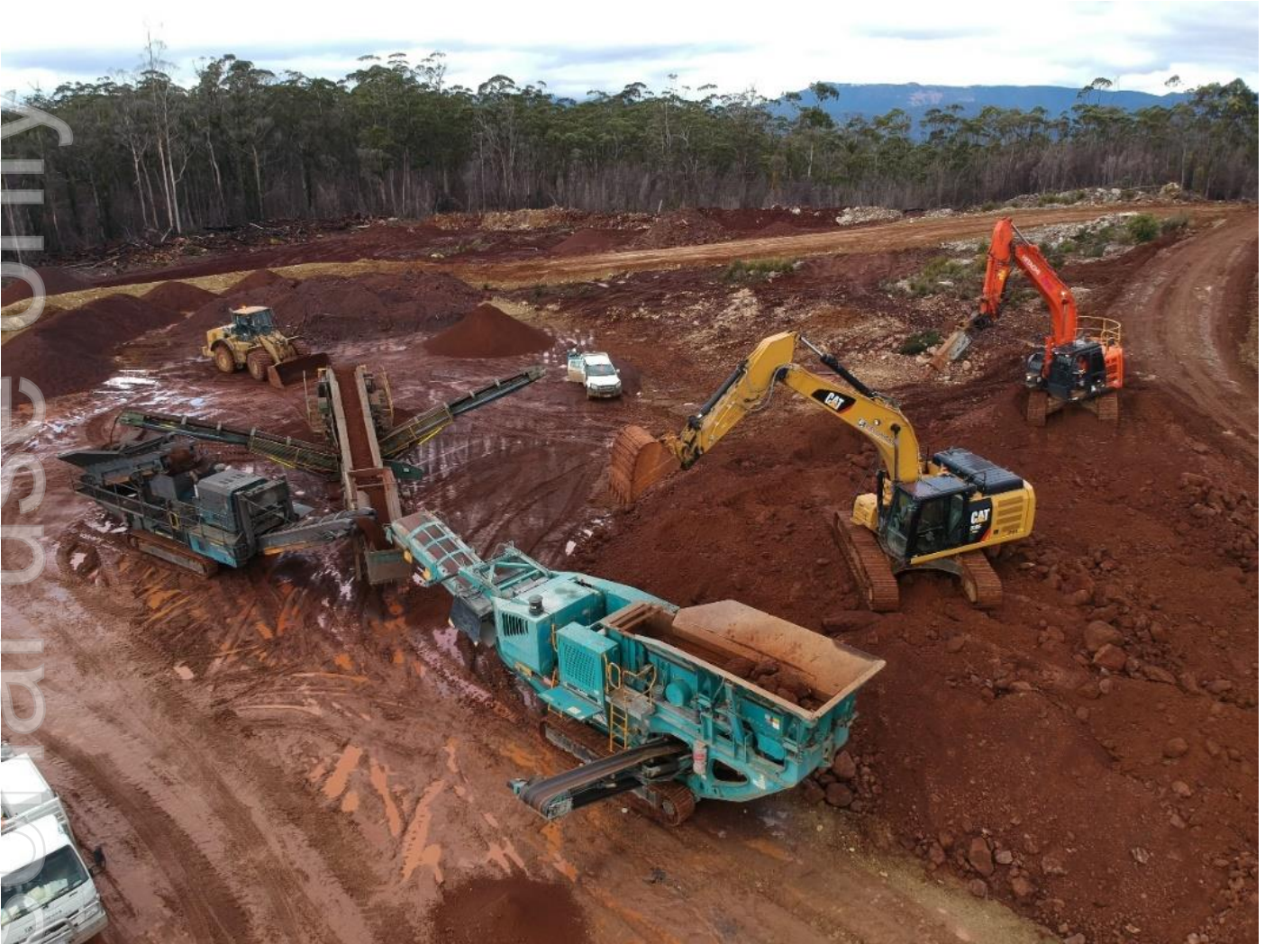
Figure 3 | Dry Screening Operations at the Riley Mine Site
