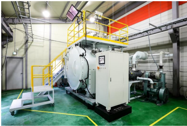
Figure 3: Ziron Tech Pilot Plant - Korea 2020
