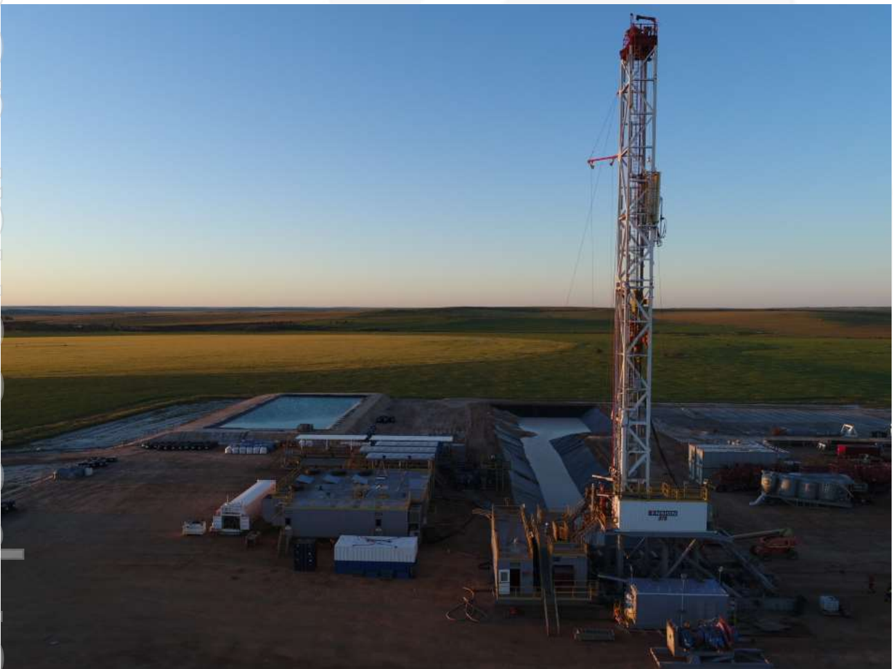
Figure 1. The Ensign 970 drilling rig at the WE-3 location.
