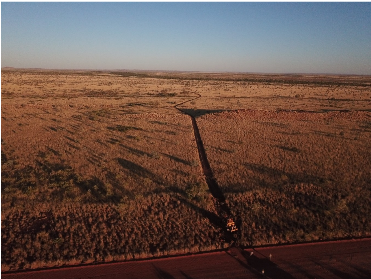
Figure 1: New access road construction commenced
