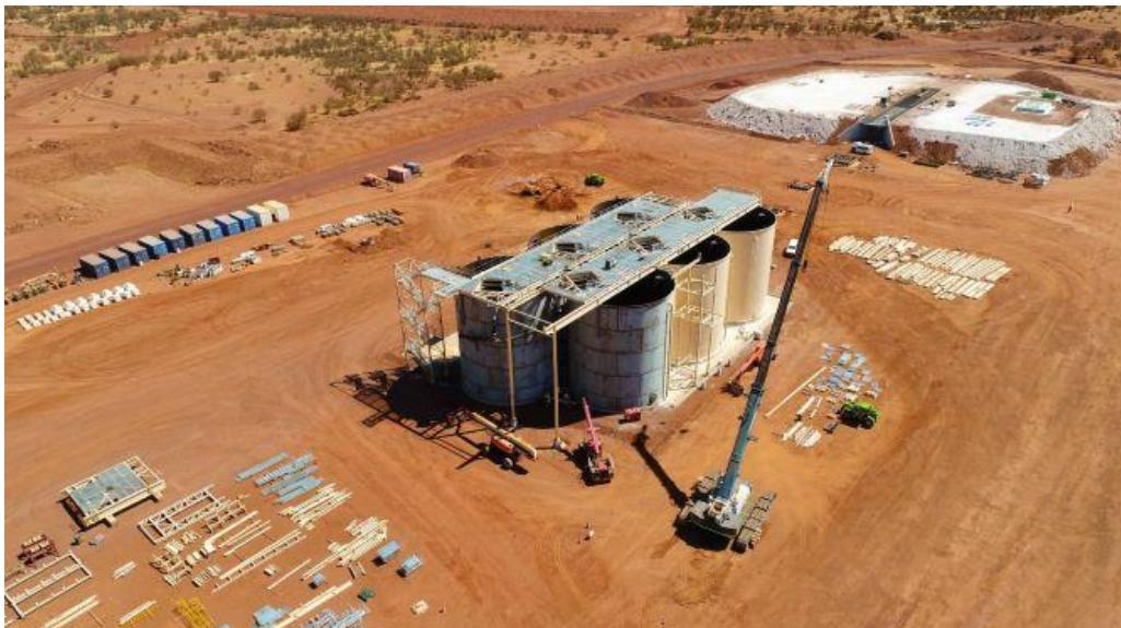
*CIL tank erection and top of tank steel installation*
