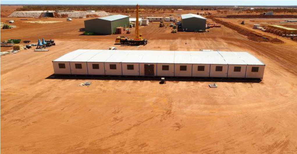
Administration office, Maintenance workshop and stores shed
