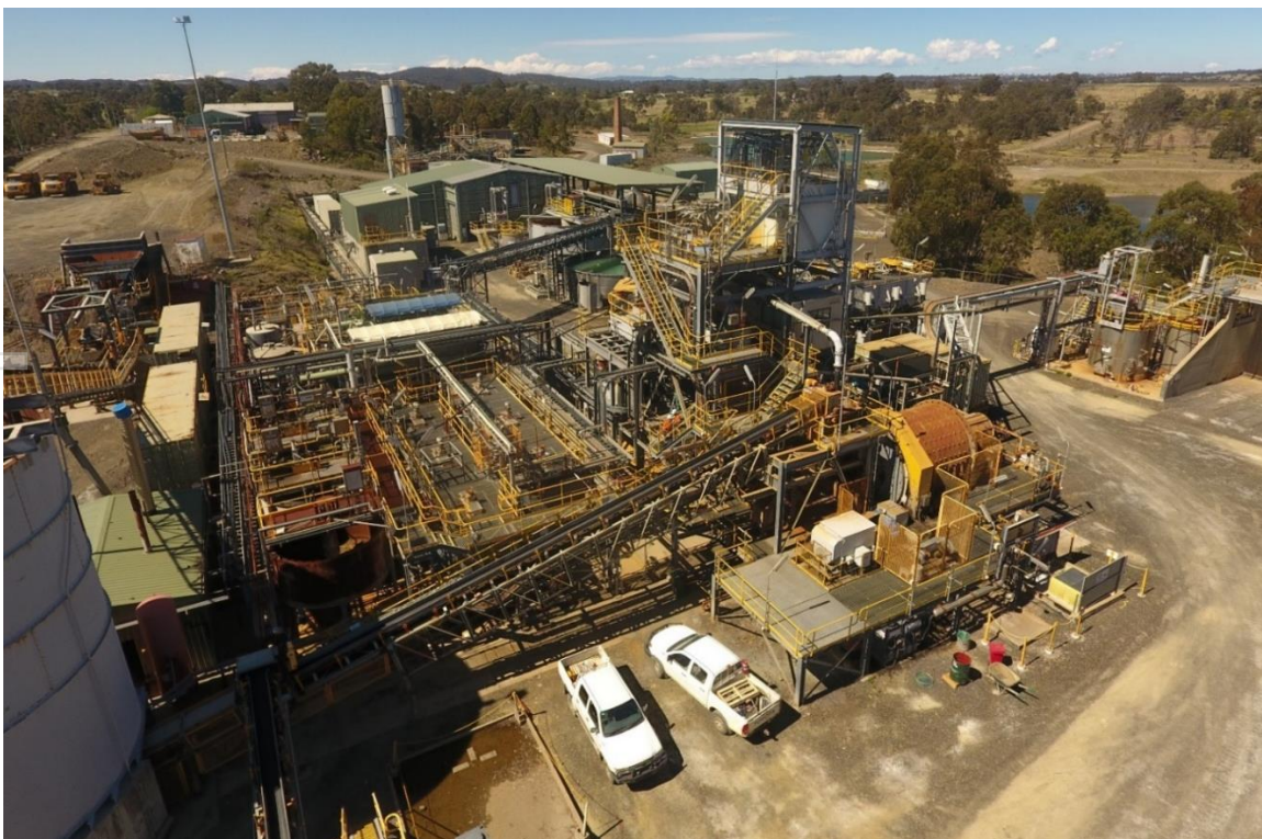
Figure 8 Hillgrove Gold Project Processing Plant
