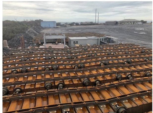
Components being prepared for Steel Pan Conveyor installation, Port Latta
