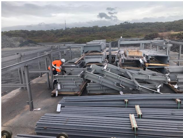
Components being prepared for Steel Pan Conveyor installation, Port Latta
