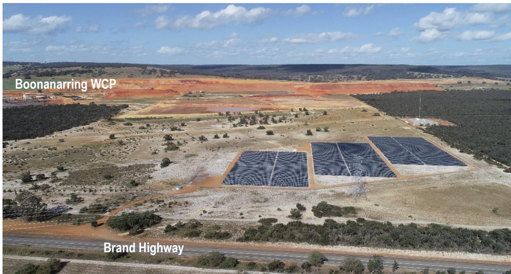
Boonanarring Solar Farm
