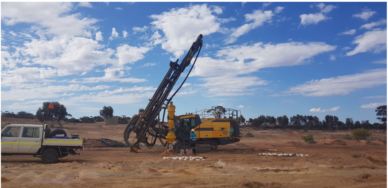
Grade control drilling ongoing
