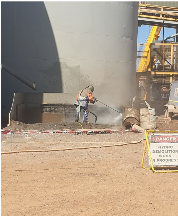
Hydro blasting ahead of concrete repair
