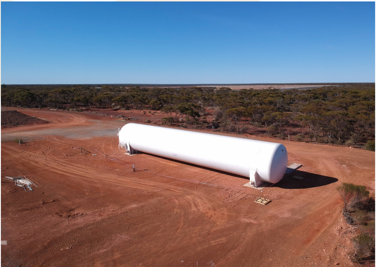
LNG gas storage bullet in position at Davyhurst
