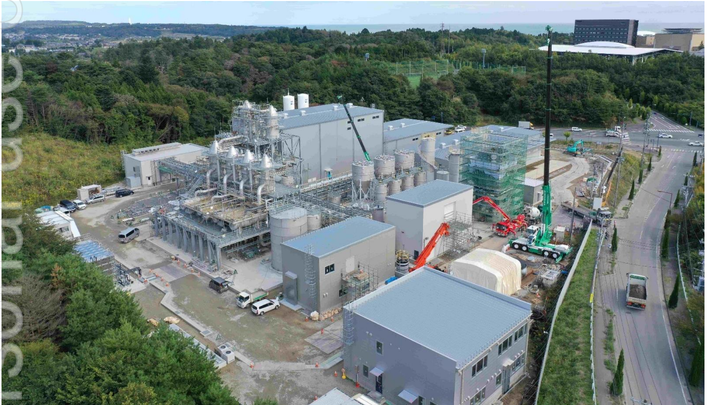
Aerial view of the Naraha Lithium Hydroxide Plant construction site
