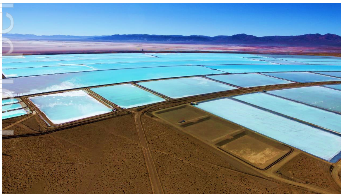
Pond construction activity
