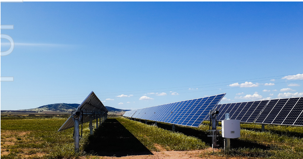
Image: A 5MW ac solar farm currently being designed and constructed by MPower
