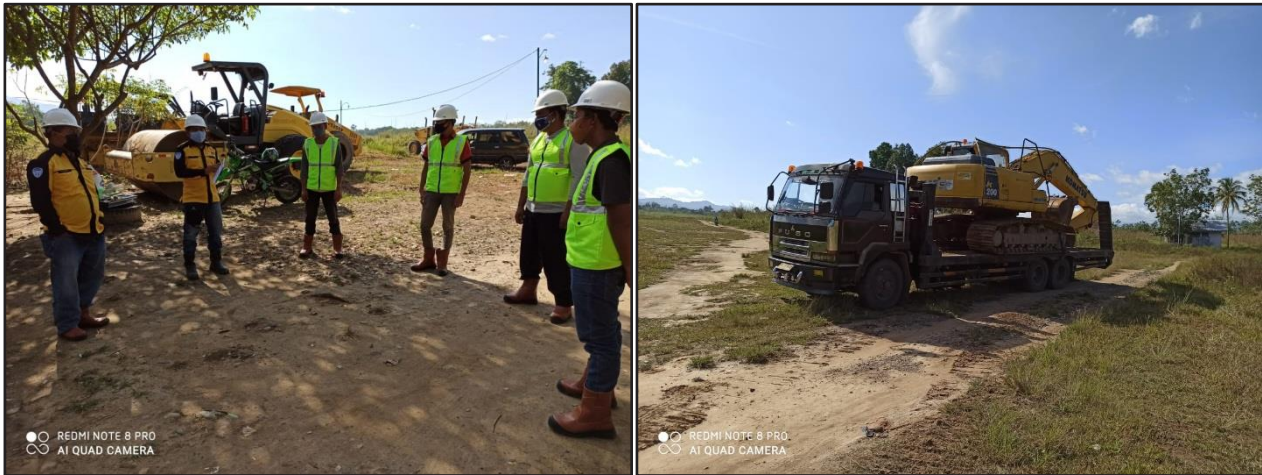
Figure 8. Sihayo Starter Project Early Works – Heavy equipment mobilization
