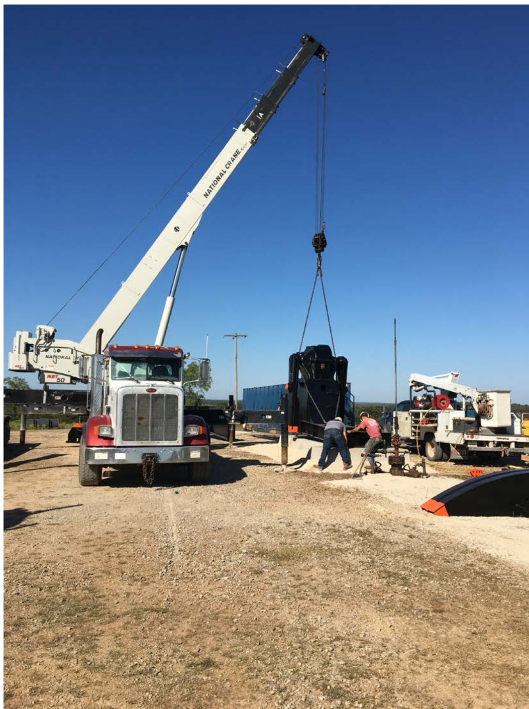
Figure 2. Production equipment being installed on the Mitchell Well in Carter County, Oklahoma
