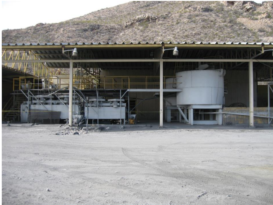
Figure 1: The Plomosas processing plant before refurbishment
