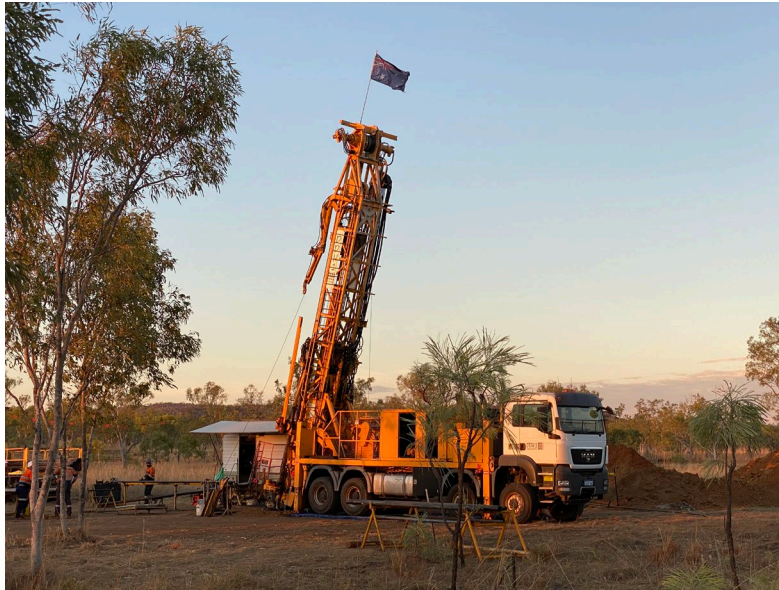
Figure 6: Diamond drilling at Merlin 29th September 2020
