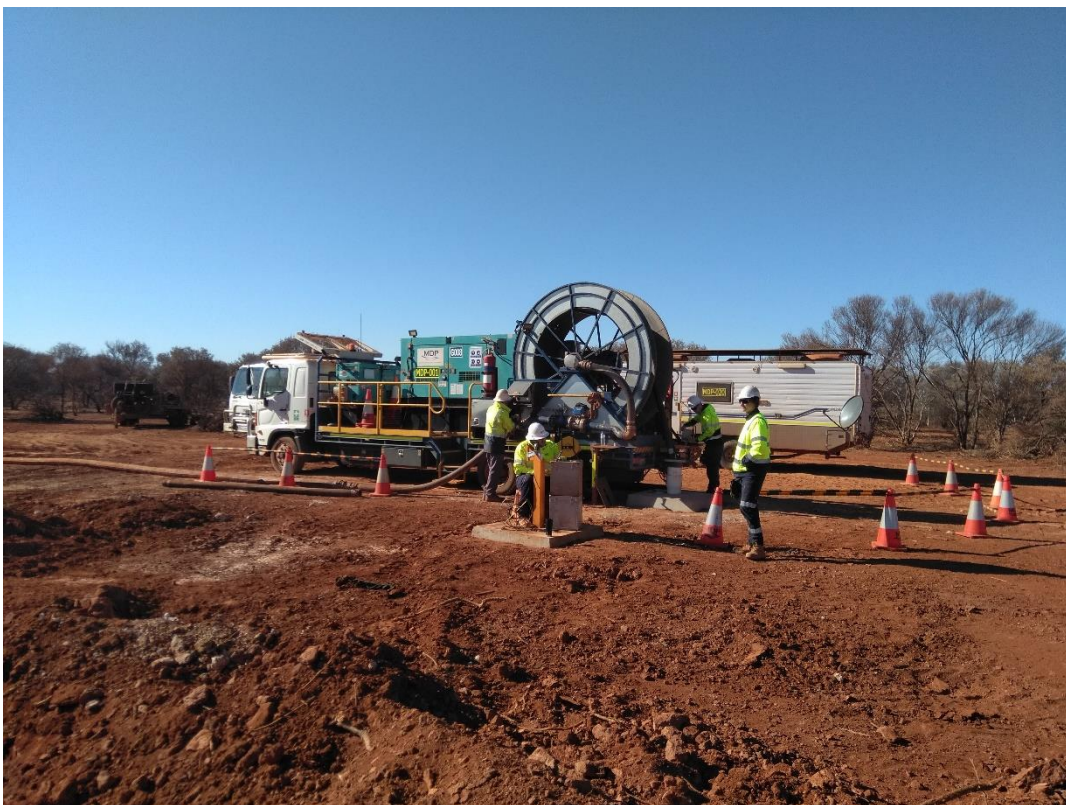
Figure 5: Water Production Bore Pump Testing
