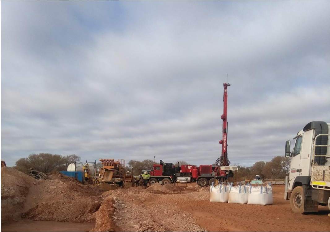
Figure 4: Water Production Bore Drilling
