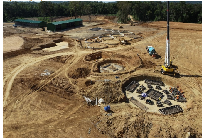
Figure Eight | Process Plant Civils
