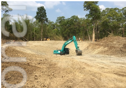
Figure Eleven | Process Plant Sediment Pond
