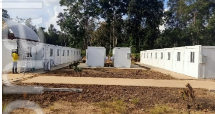
Figure Four | Village Construction Works
