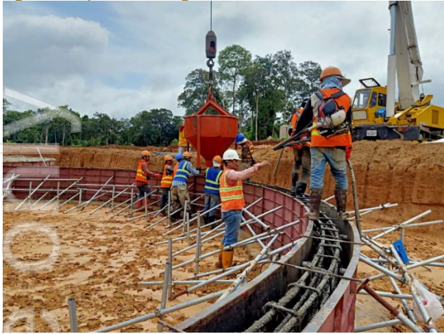
Figure Nine | CIL Tank Ring Beams
