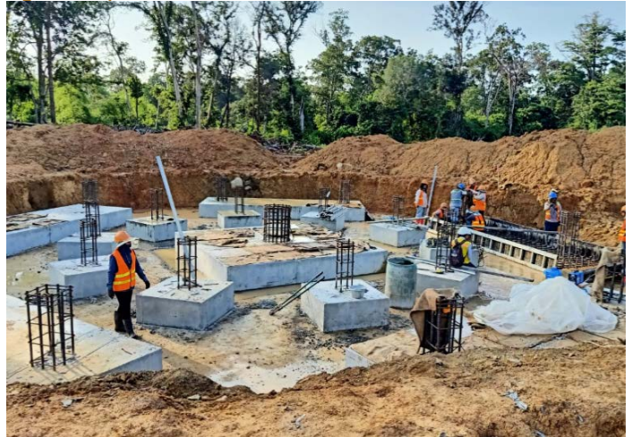
Figure Ten | Float Cell Foundation
