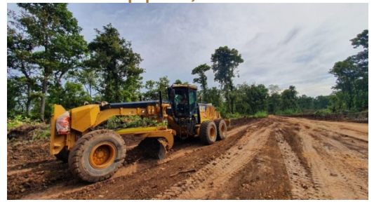
Figure Thirteen | Contractor Yard Clearing (MACA Commissioned Equipment)
