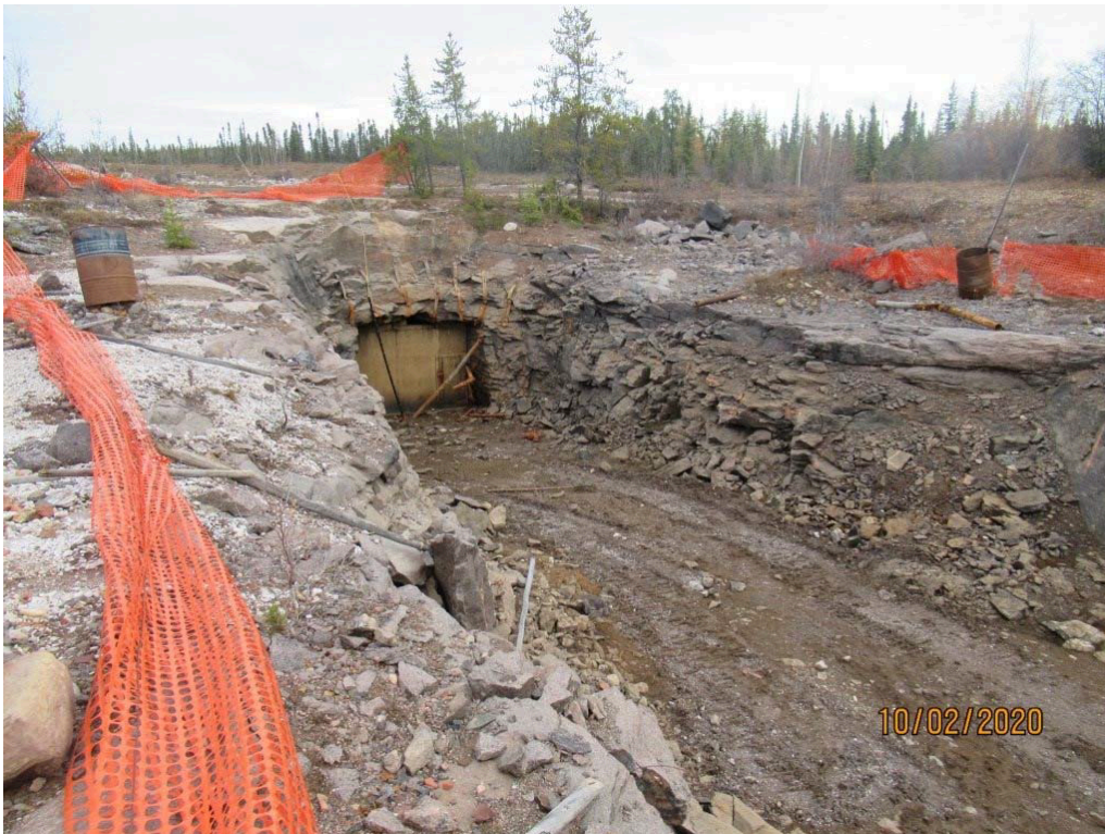
Figure 2: Nechalacho decline dewatered
