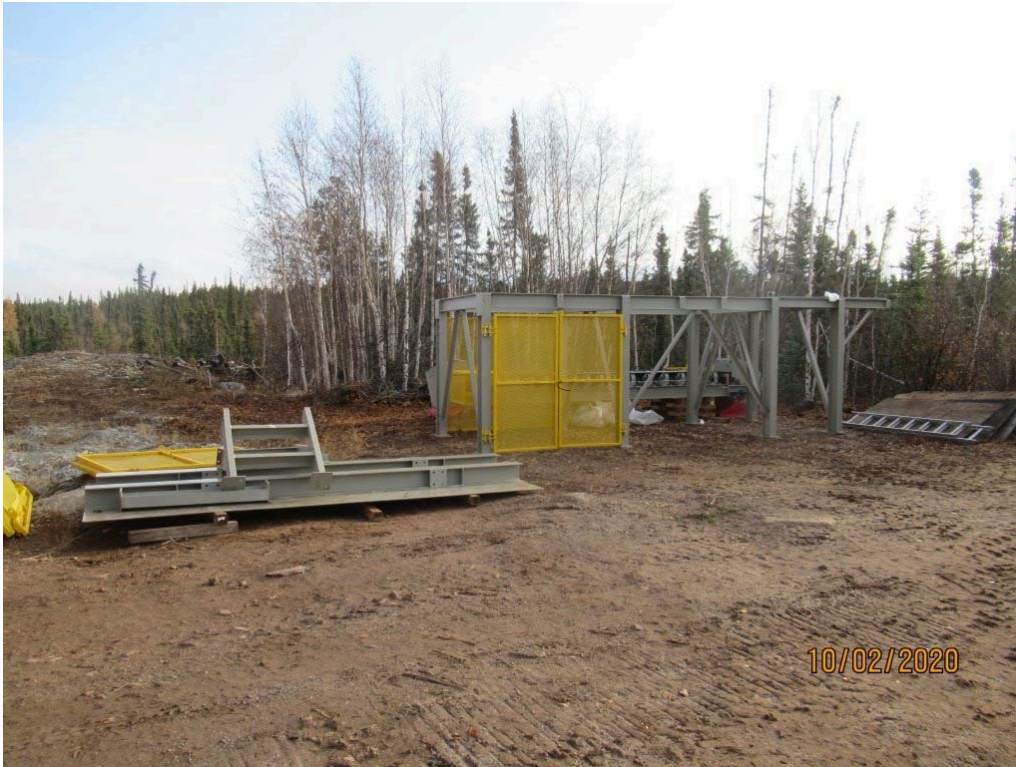
Figure 1: Ore sorter base and substructure delivered to site
