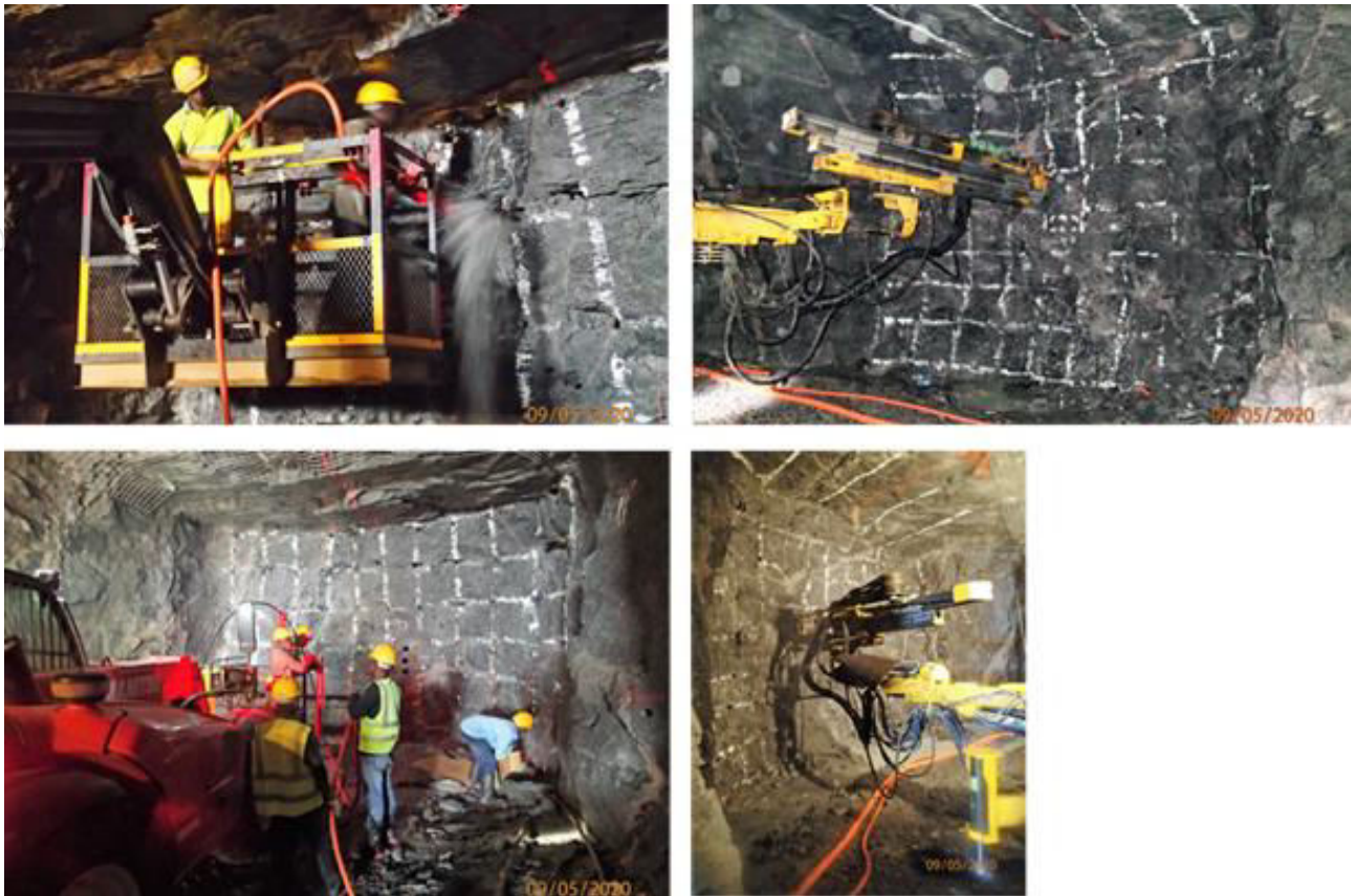
Figure 2: Underground drill and blast work underway. Top right and bottom right: drilling blast holes on a regular grid pattern; Top left: cleaning drilled holes; Bottom left: charging blast holes.
