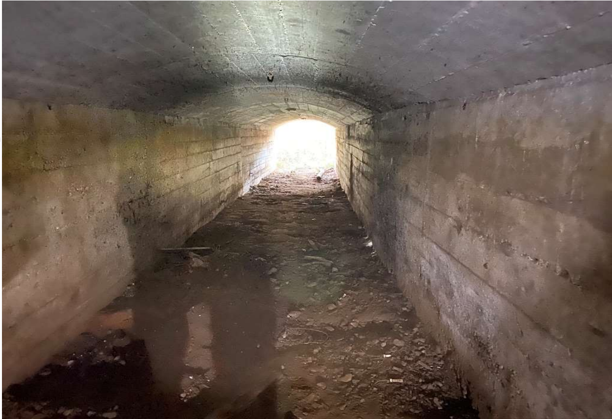
Figure 11: Clewer Dukes Morgons Mine Access Portal
