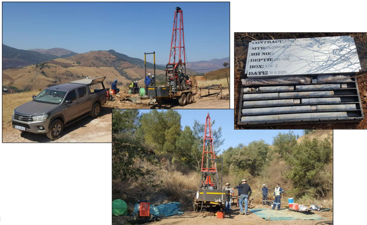
Figure 1: Triple core diamond drill rig collecting orientated core for engineering studies
