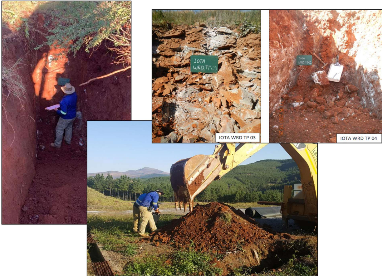
Figure 2: Test pits for ground stability
