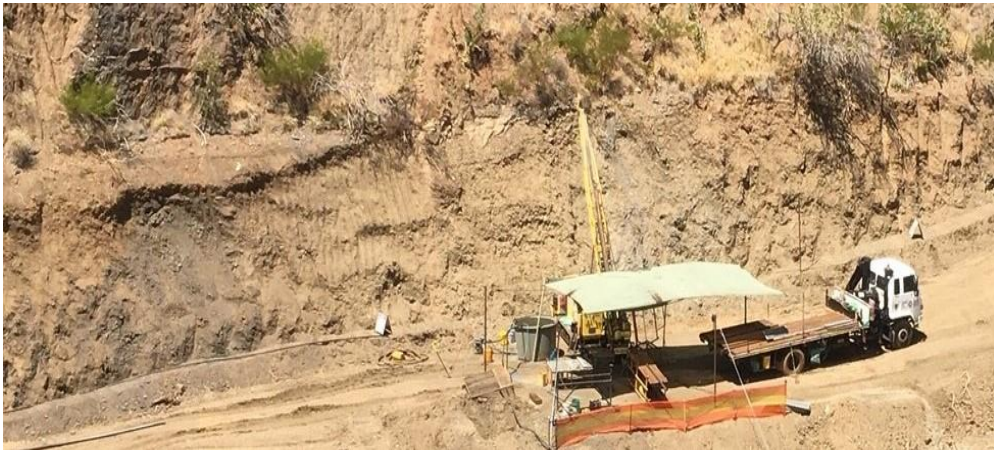
Figure 1: Upgrade Resource drilling on the decline in the Mt Freda pit.
