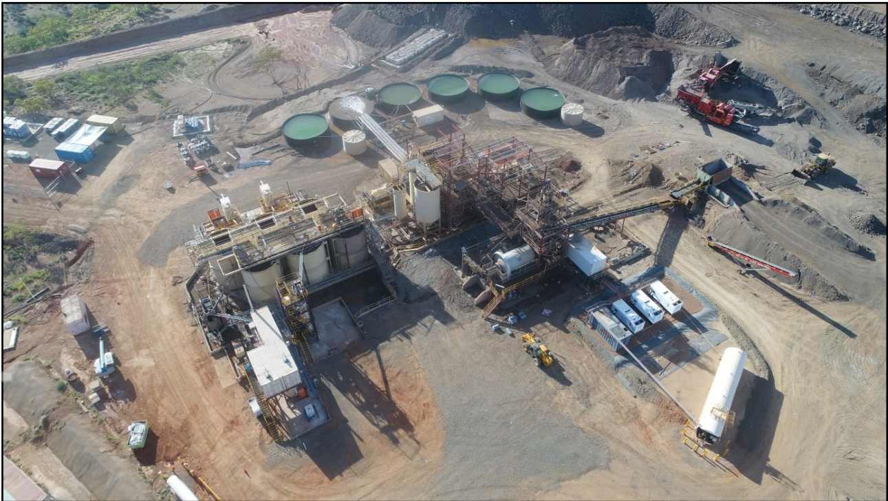
Lorena Gold Mine CIL Processing Plant
