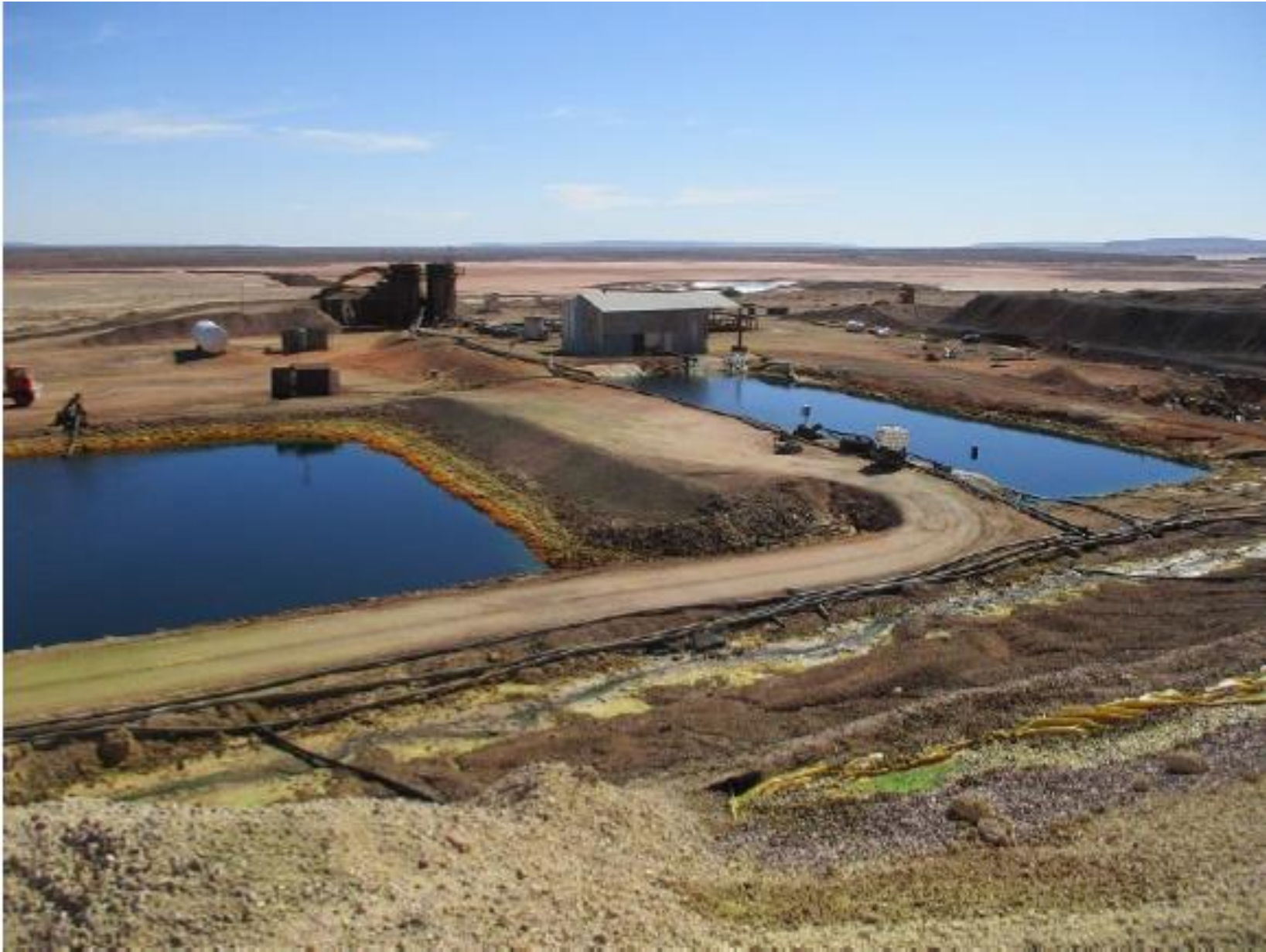
Figure 13: View of Mt Gunson Oxide Treatment Facilities and Leach Ponds, 2019
