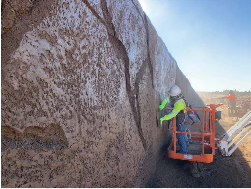
Figure 2. Carving the concrete to replicate a rock face
