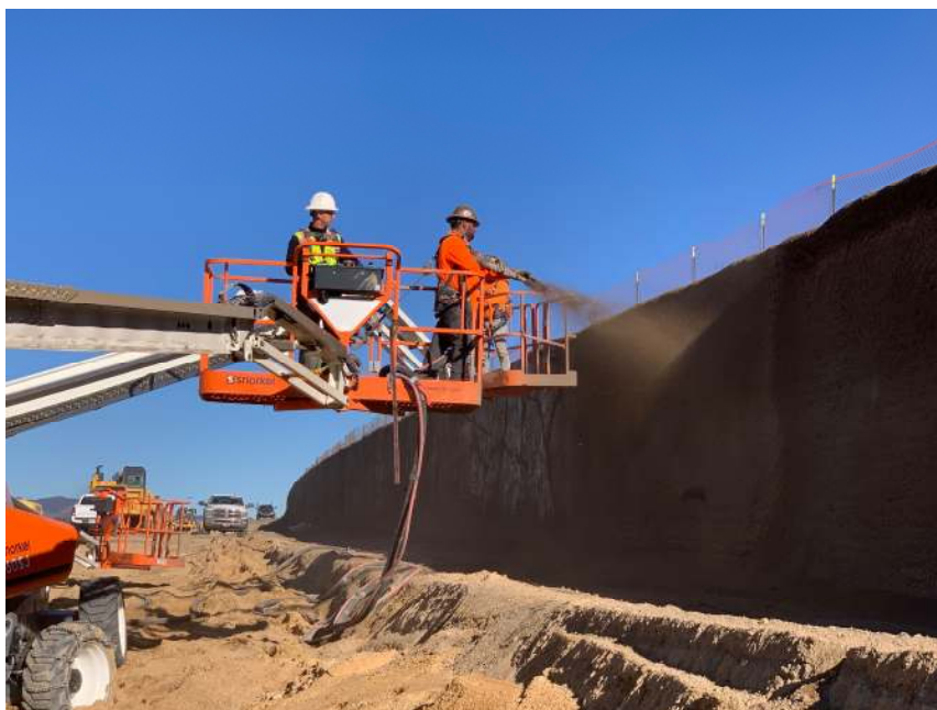
Figure 1. Applying the shotcrete to the wall along I-20 at Colorado Springs
