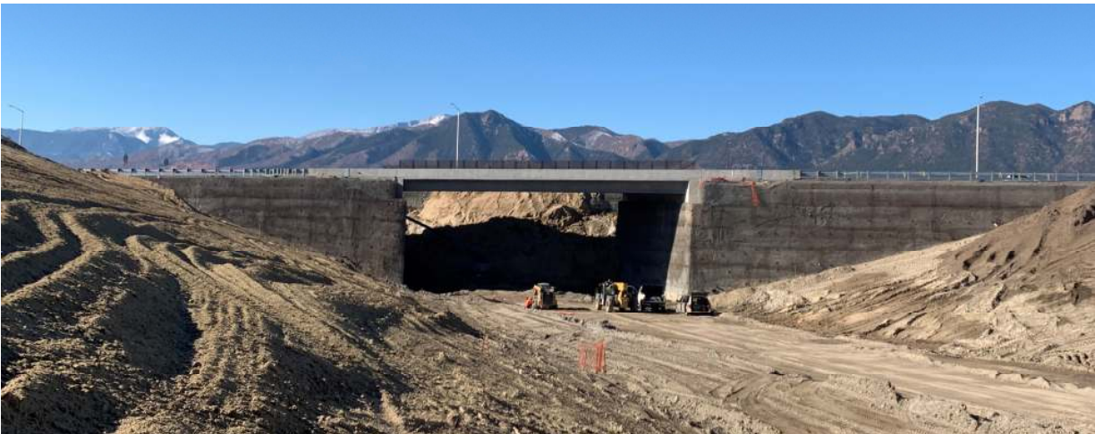
Figure 3. Underpass, wing walls and embutment constructed with EdenCrete® enriched concrete
