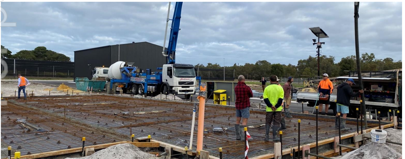
Photographs of commencement of slab pour for ClearVue greenhouse at Murdoch.
