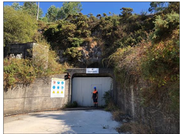
Figure 4.5 Portal to the ramp of Santa María, northeast of Mina Carmen.
