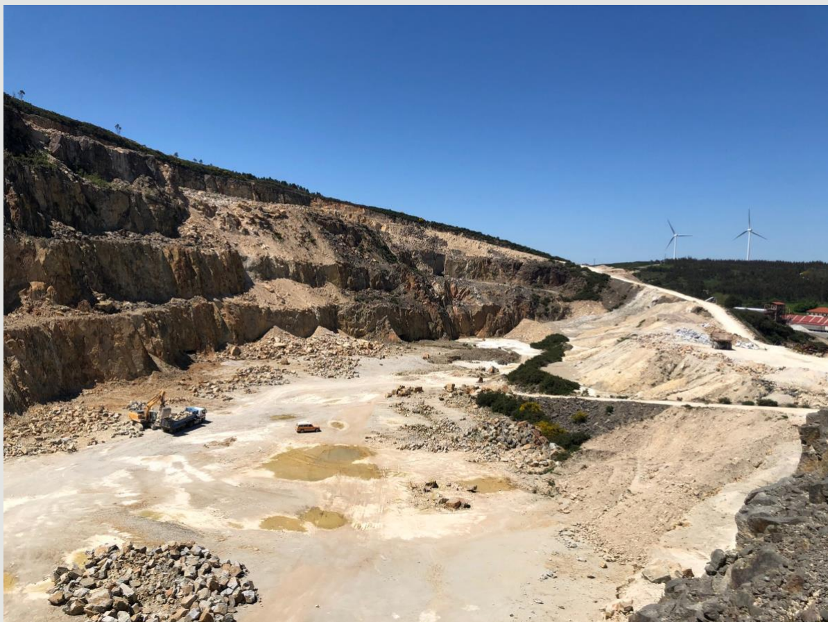
Figure 6.1 North and west walls of Santa Comba quarry
