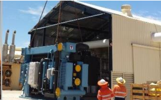
Installation of Absorption chiller
