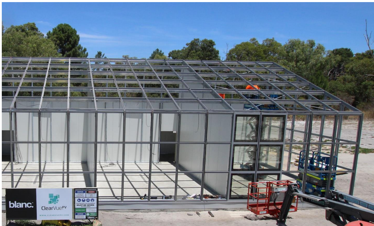
Photographs of commencement of glazing onto ClearVue greenhouse at Murdoch.
