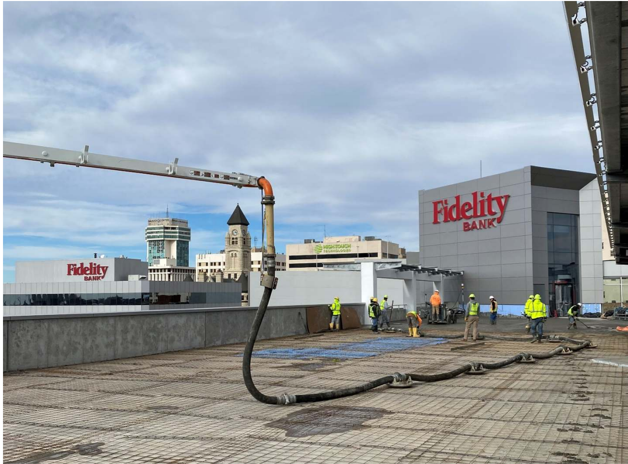
Figure 6. Installing top deck of car park
