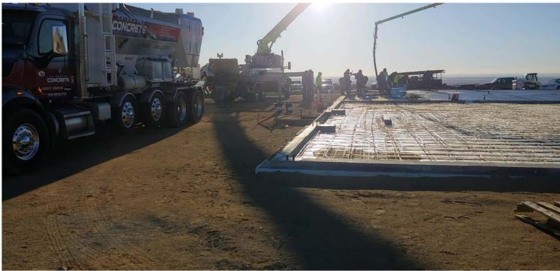
Figure 3. Volumetric truck mixing at the Loveland project site
